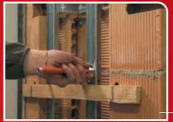
Insert the fixing pivots at the desired height.
