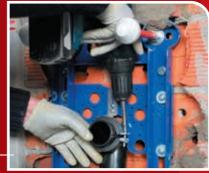
Fix the drain pipe on the pipe clamp and adjust it in height.
