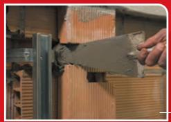
Fix the bracket with a wooden crossbeam and wall it in through its shaped ends.
