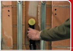
Set drain pipes and water supply pipes - for either toilet bowl or bidet in the right place. Wall the bracket in.
