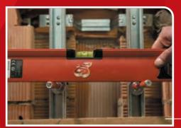
Level the fixing pivots.
