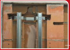
Make the breaks in the masonry, fit the bracket in and level it.
