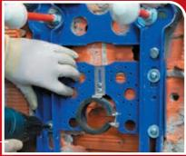
Adjust the plate in height if necessary.
